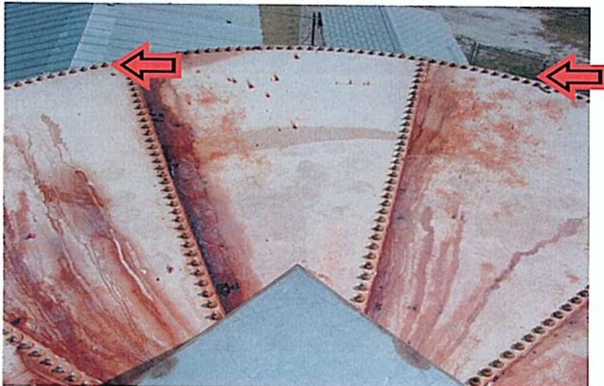
Photo shows the tank roof is not equipped with an OSHA required fall protection system. We recommend installing an approved 42" high handrail system around the circumference of the tank roof, complete with toeboard, intermediate rail and a stainless steel gate chain at the junction of the shell-to-roof access ladder and tank roof as required by OSHA (see glossary).
