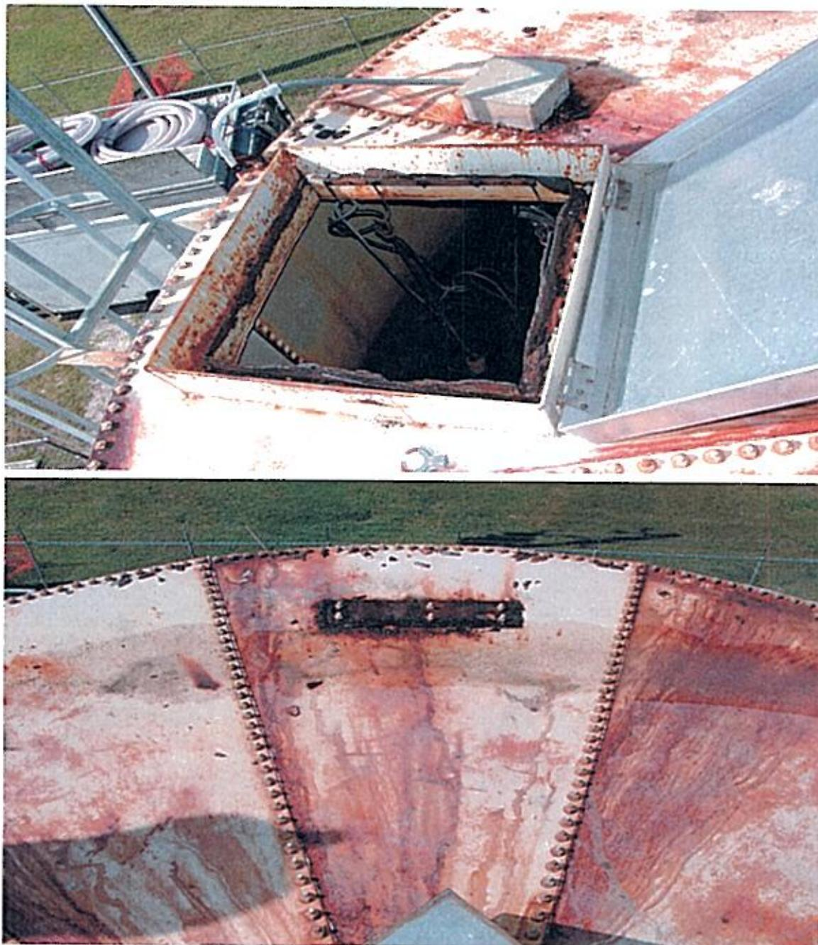
Photos show the condition of the exterior paint system. We recommend sand-blasting the tank exterior to an SSPC #6 (commercial) blast, apply one (1) full coat of primer, then applying one (1) finish coat of Alkyd.
